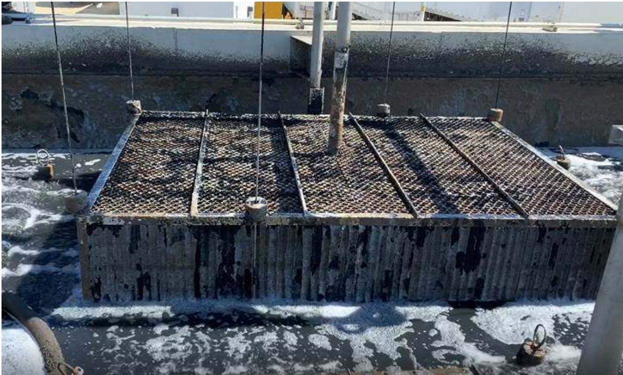
*Figure 3: Retrievable BIOcube unit*
